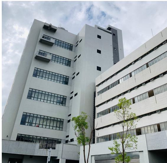
Figure4-2 The new pharmaceutical building for controlled drugs
