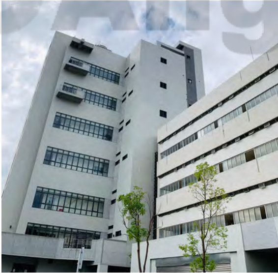
Figure 4-1 New manufacturing facility for controlled drugs
